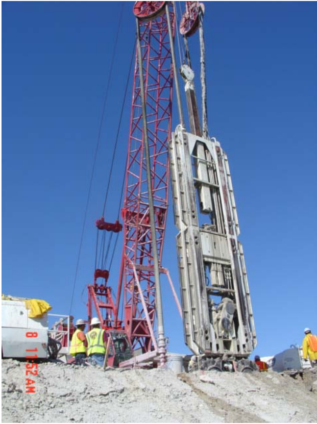
Figure 1. Hydromill being extracted from cut-off wall trench, at Herbert Hoover Dike, FL (Courtesy of TREVIICOS South).
