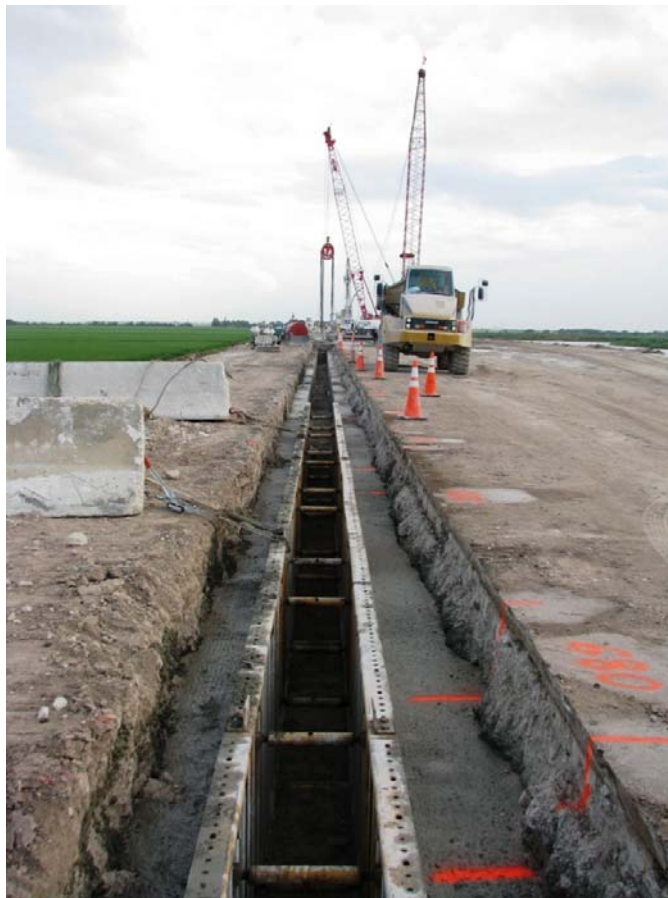
Figure 5. Guide wall for remedial cut-off wall
