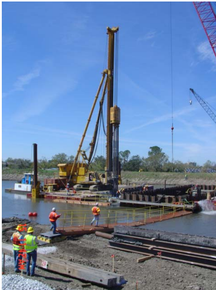
Figure 2. DMM machine (triple axis) operating in levee conditions, New Orleans, LA (courtesy of Raito Inc.).
